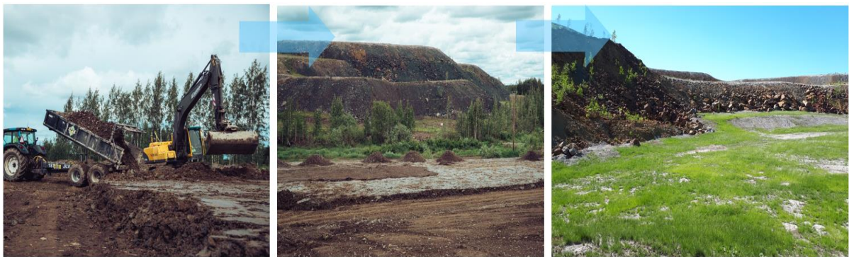
Figure 8. Clay cover structures construction from left to right towards finished structure.
